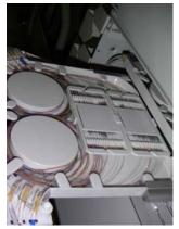
The incoming fiber is always the fiber going towards the NCAR/UCAR Mesa lab site. The outgoing fiber is the cable going towards the NCAR/UCAR Foothills lab site. However there is an exception at the CU Telecom location where the top panel goes to the City Atrium building and the bottom panel goes to CU Engineering.
